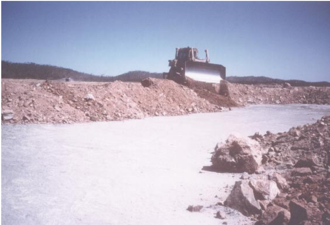
Figure 12 A tailings dam being capped. Environmental management of mine sites is the best it has ever been.
