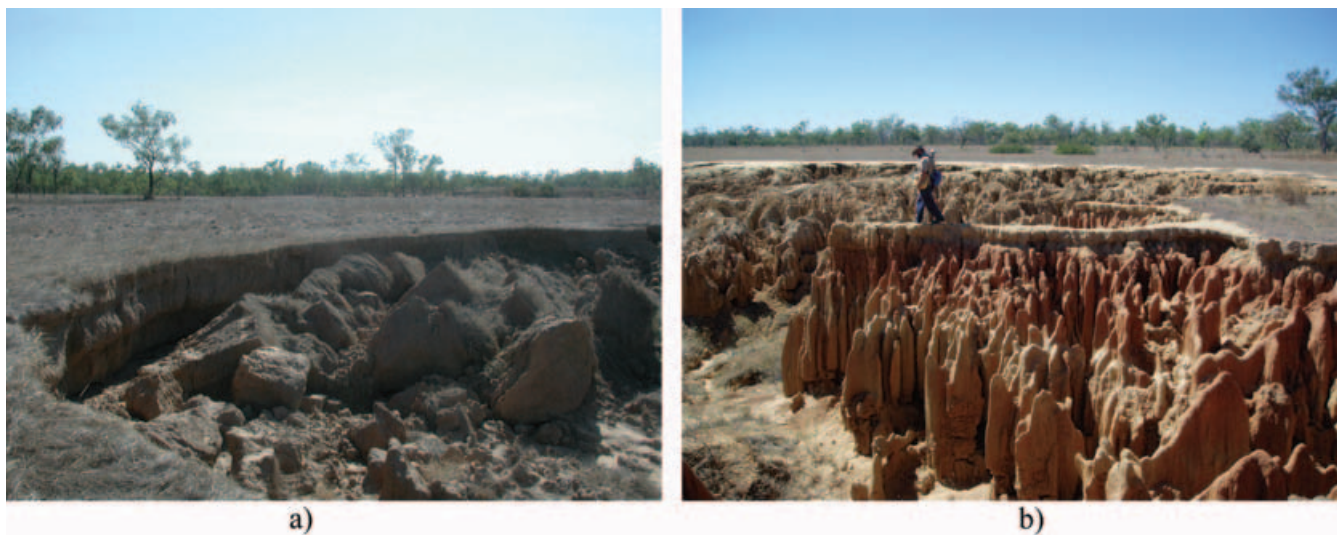
Figure 11. Ground photographs of (a) mass failure, and (b) fluting and carving at head scarps.
